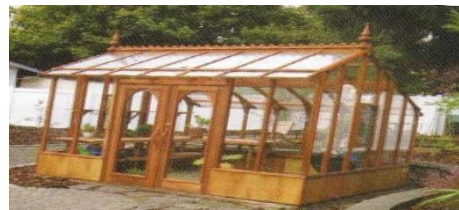
8- Gable uneven span
